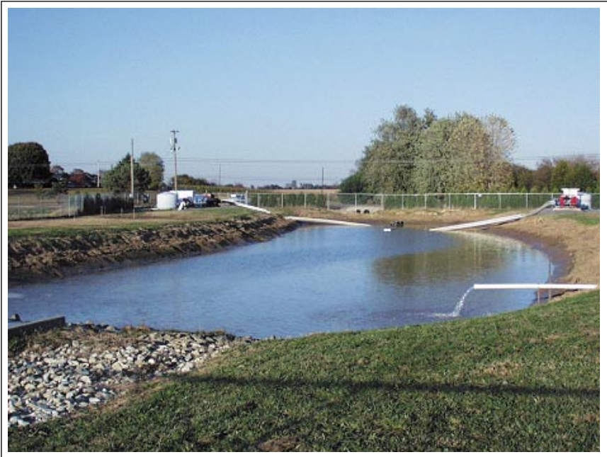
Figure 4. Finished tailwater recovery system.
