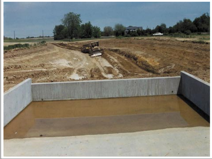
Figure 1. Concrete catch basin.
